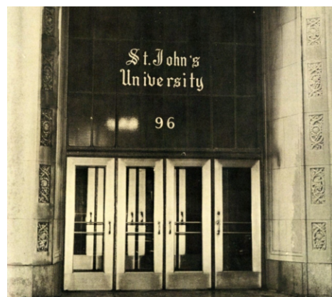
Entrance to 96 Schermerhorn Street.
